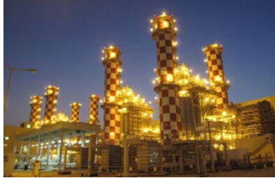
• Al Dur Power Plant
