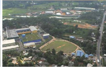
Kelani Right Bank WTP to be Upgraded
