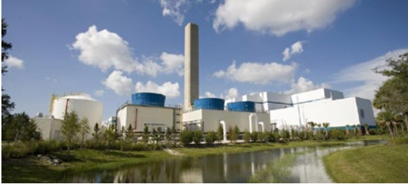
• Lee County Waste-to-Energy Plant
