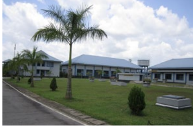
Kandana WTP to be Upgraded
