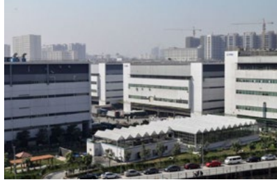
Shenzhen IFFAS Plant
