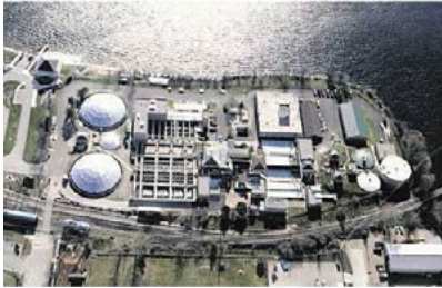
Michigan MBR Plant
