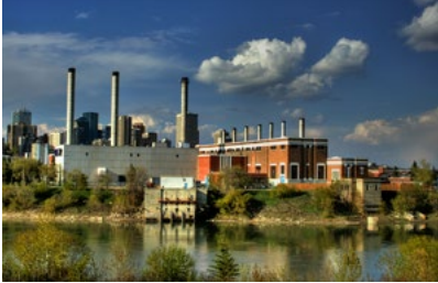
• Rossdale Power Plant
